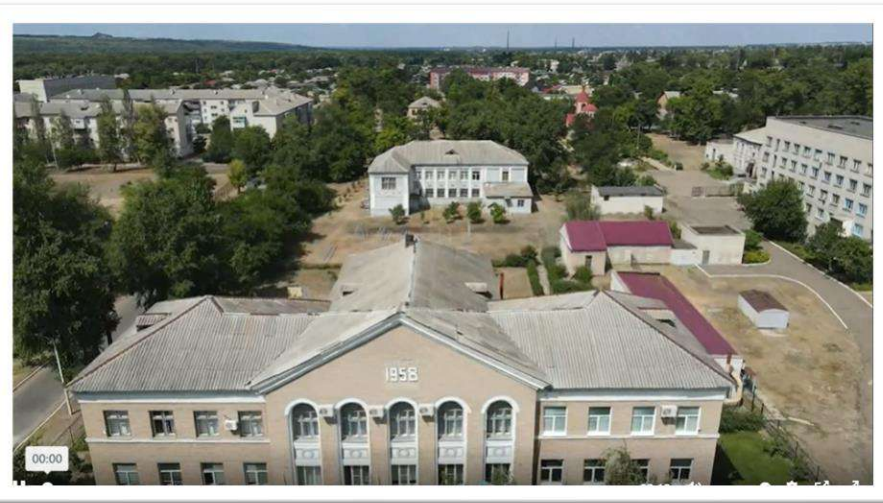
Rubizhne Vocational Chemical-Technological Lyceum. Replacement the roof.
